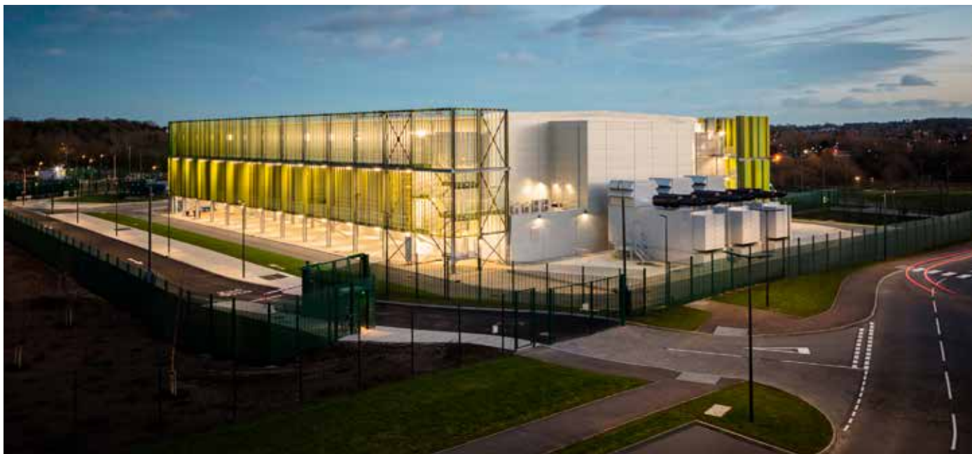
▼ Modern data centre facilities
